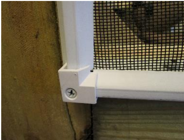
Photo No. 3 Corner Bracket Installation
